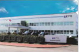
Fábrica de Dalian (China) Aparamenta MT/BT, contactor MT Aparamenta MT/BT, Mould TR
